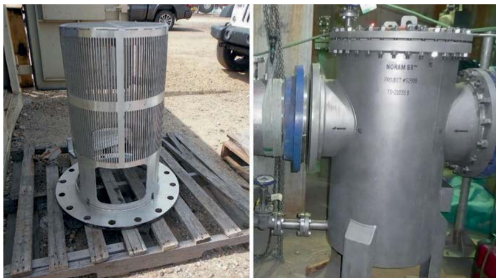
Fig. 5: Acid strainer. Project A (left): internal strainer. Project B (right): external strainer.
