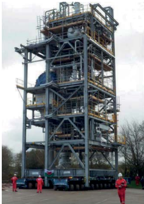
Fig. 3: Transport of converter module with SPMT.
