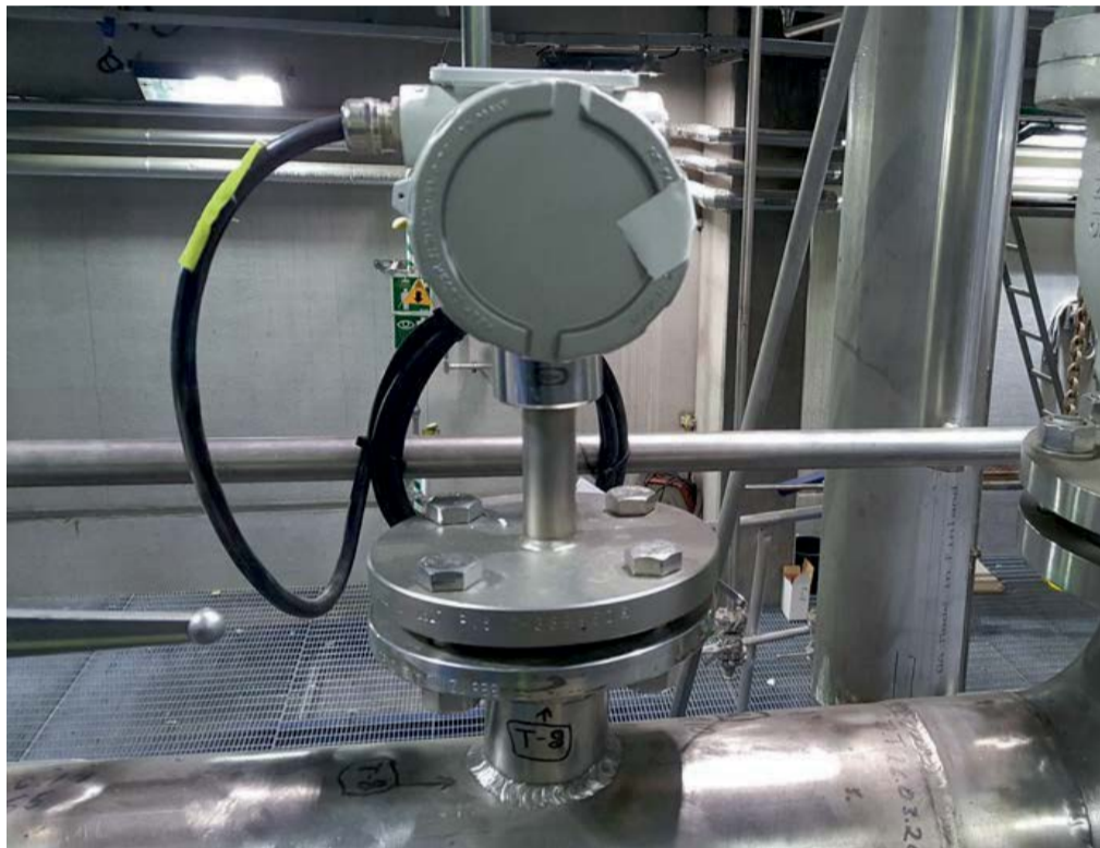
Fig. 2: LiquiSonic® inline immersion sensor.
