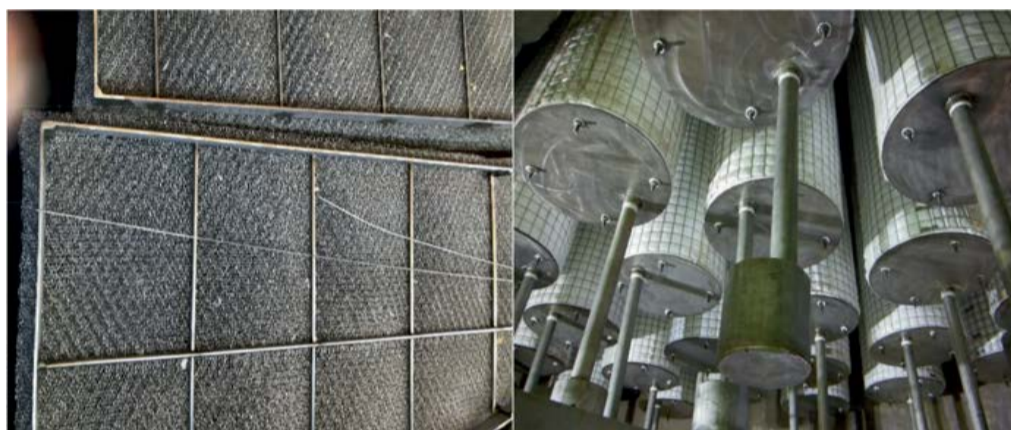
Fig. 3: Mist Eliminators. Project A (left): mesh pads. Project B (right): Brownian diffusion candles.
