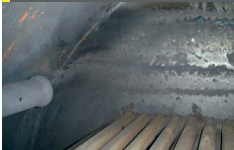
Fig. 9: Inlet tubesheet with continuous blowdown collection
