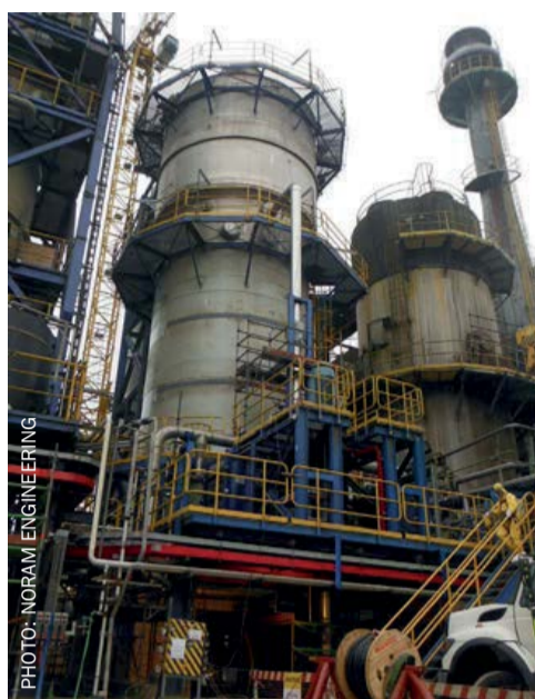
NORAM acid tower installation at a Codelco plant in Chile.
