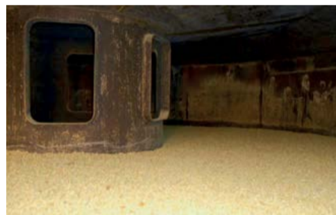
Fig. 3: Reactor bed of Quattro catalyst.
