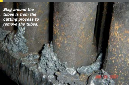
Fig. 10: FAC corrosion on bottom of tubes at the hot gas inlet
