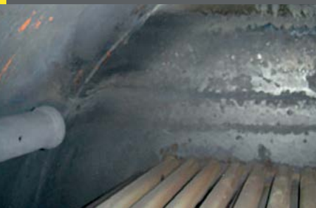
Fig. 9: Inlet tubesheet with continuous blowdown collection
