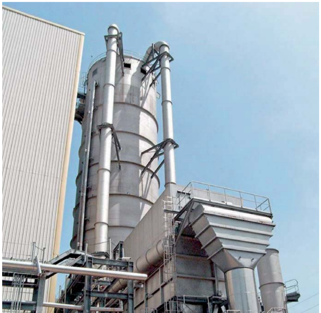
Fig. 1: Example of a modern prilling tower.
