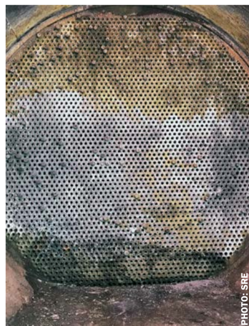
Fig. 3: Condenser bed – tube view.
