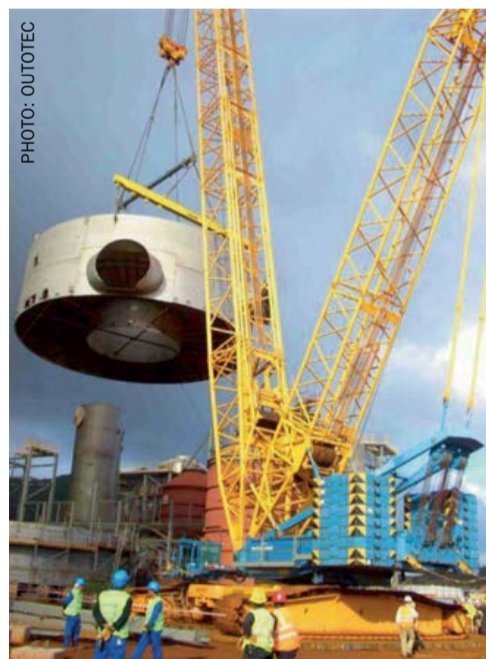
Fig. 8: converter construction at site.
