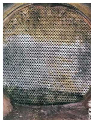
Fig. 3: Condenser bed – tube view.
