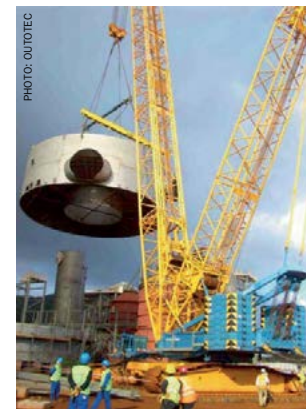
Fig. 8: converter construction at site.
