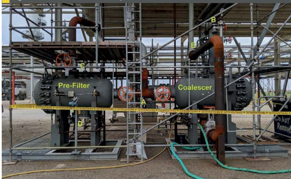
Fig. 5: Installation at the refinery
