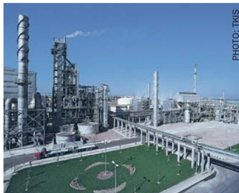
Abu Qir 3 plant, Egypt.
