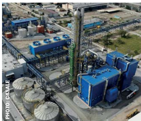
Fig. 2: JSC Navoiyazot nitric acid plant.
