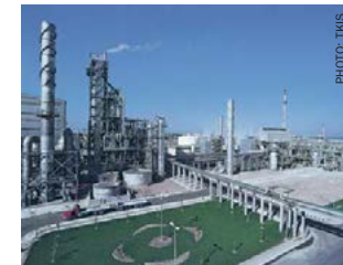
Abu Qir 3 plant, Egypt.
