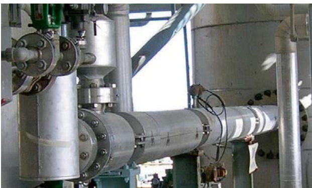
Fig. 5: Casale pipe reactor.
