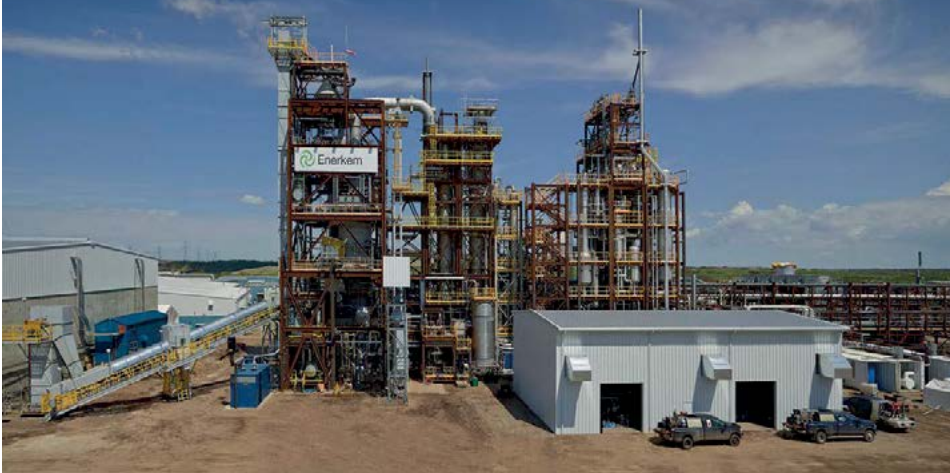
Enerkem's municipal waste gasification plant at Edmonton, Alberta.
