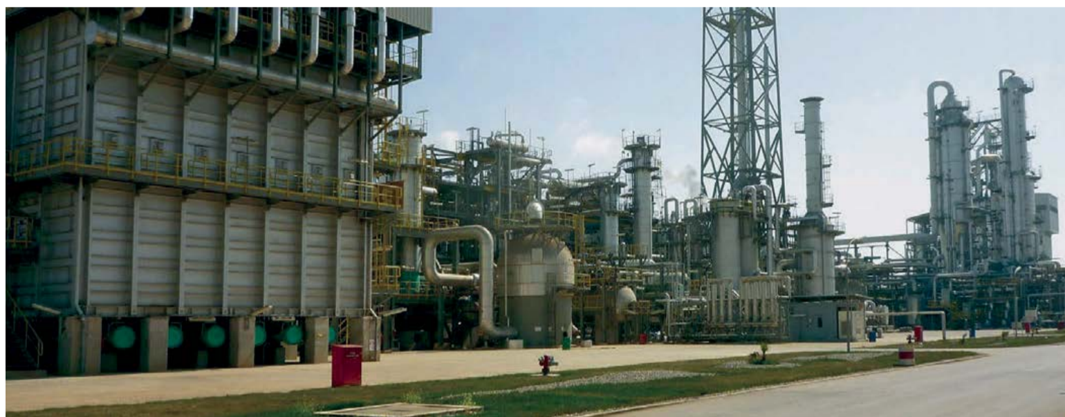
Steam methane reformer (left) in an ammonia plant.
