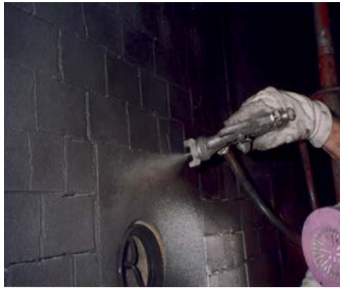
Fig. 14: Ceramic coating application on refractory brick lining.
