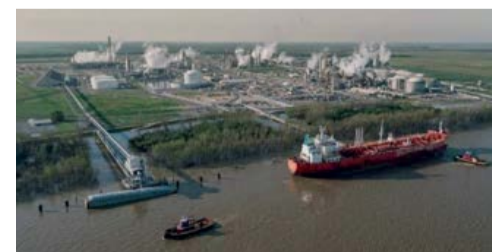
CF Industries' nitrogen complex at Donaldsonville, Louisiana.
