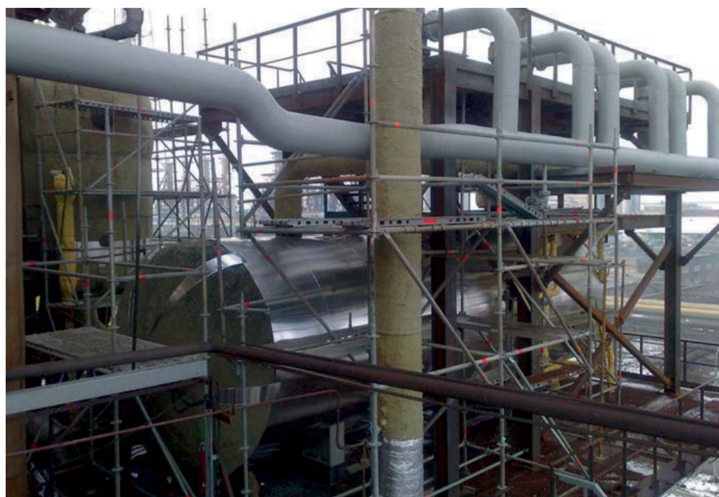
Fig. 8: Pre-desorption unit installed in a GIAP ammonia plant.
