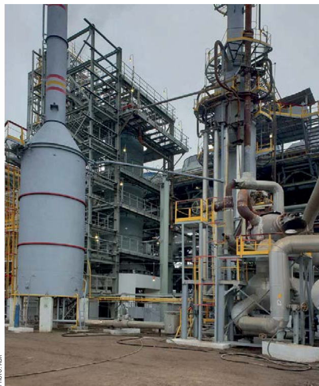
Fig. 4: Add-on ammonia converter.
