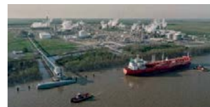
CF Industries' nitrogen complex at Donaldsonville, Louisiana.
