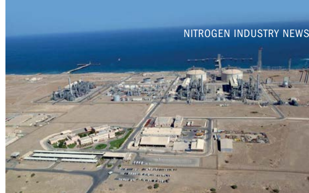
The Omifco urea facility (left), next to the Oman LNG complex at Sur.
