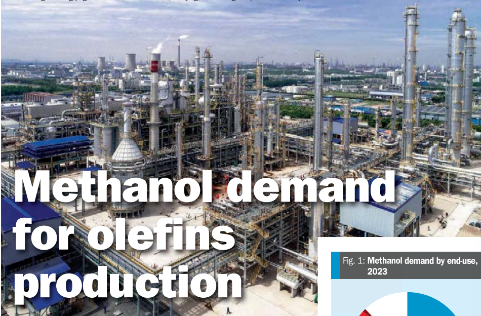
The Chengzhi Yongqing methanol to olefins unit, Nanjing, which began operations last year.
