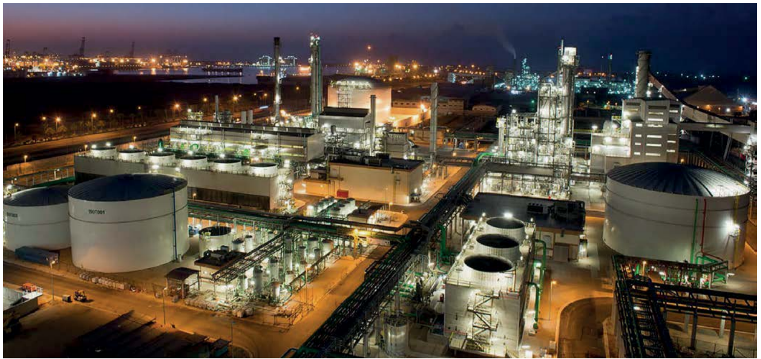
Fig. 3: ENPC ammonia/urea complex (view by night on train 1 including ammonia storage tank and the adjacent new Damietta harbour).
