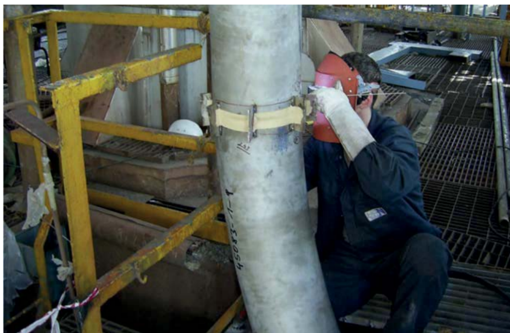
Fig. 6: SBN welder working on site.
