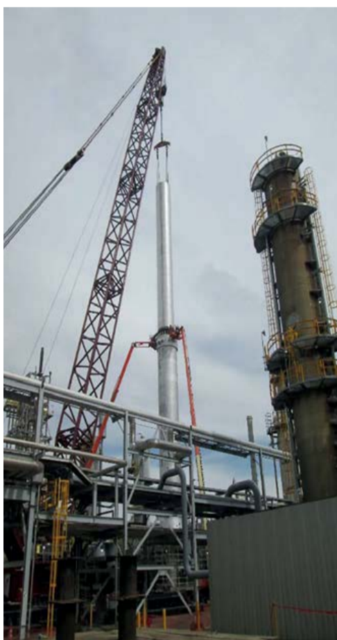
Fig. 7: Cartridge lift and installation inside converter.
