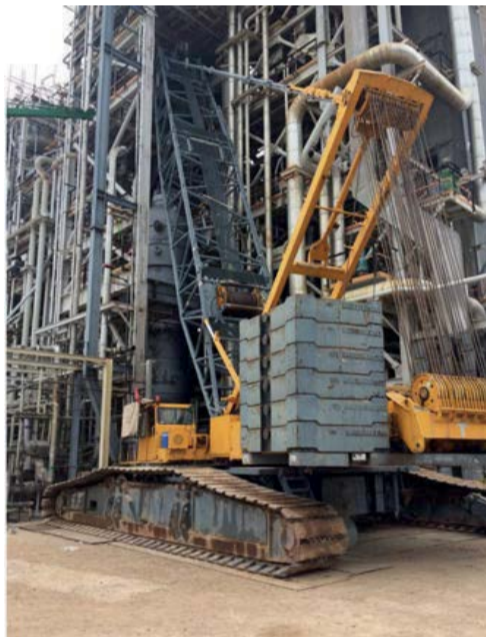
Fig. 12: Opening in steel structure allowing access to the HP stripper.
