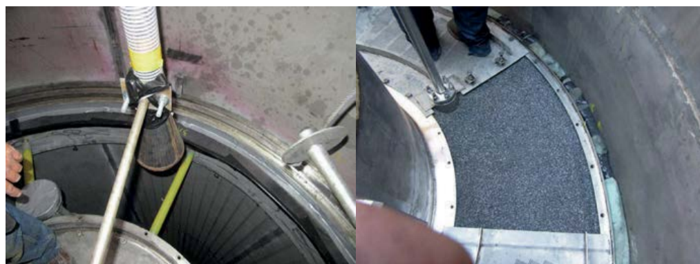
Fig. 9: Catalyst dense loading.
