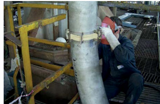
Fig. 6: SBN welder working on site.
