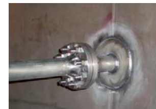
Fig. 15: Installed radar stand pipe – view from inside the vessel.
