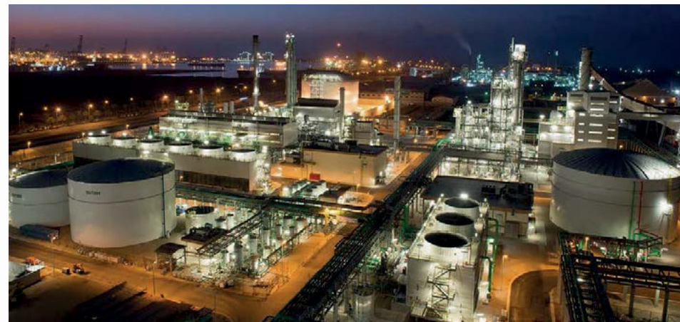
Fig. 3: ENPC ammonia/urea complex (view by night on train 1 including ammonia storage tank and the adjacent new Damietta harbour).
