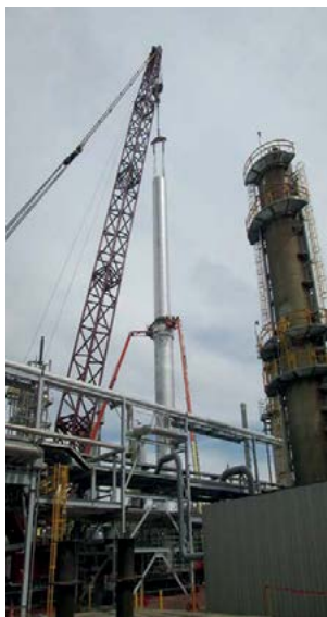
Fig. 7: Cartridge lift and installation inside converter.
