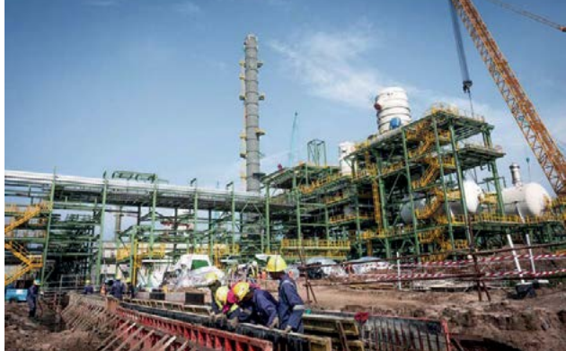
The new Dangote fertilizer complex under construction.
