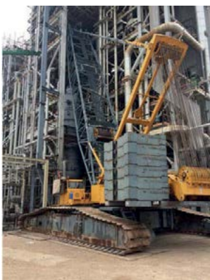
Fig. 12: Opening in steel structure allowing access to the HP stripper.
