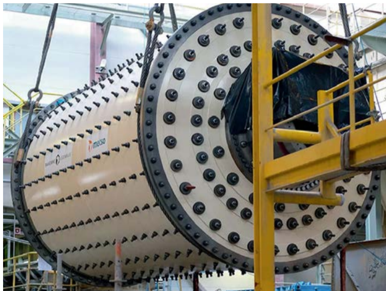
A new Metso Outotec grinding mill being lowered into place with millimetre precision at Yara's phosphate concentration plant in Siilinjärvi, Finland.
