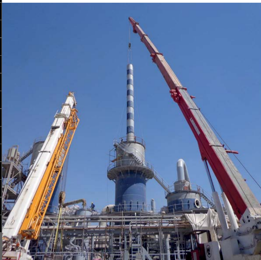
Left: The new tower as it is lifted into place at Unit 6. Right: Since start-up, Unit 6 has operated to performance guarantees, producing up to 640 t/d of acid.
