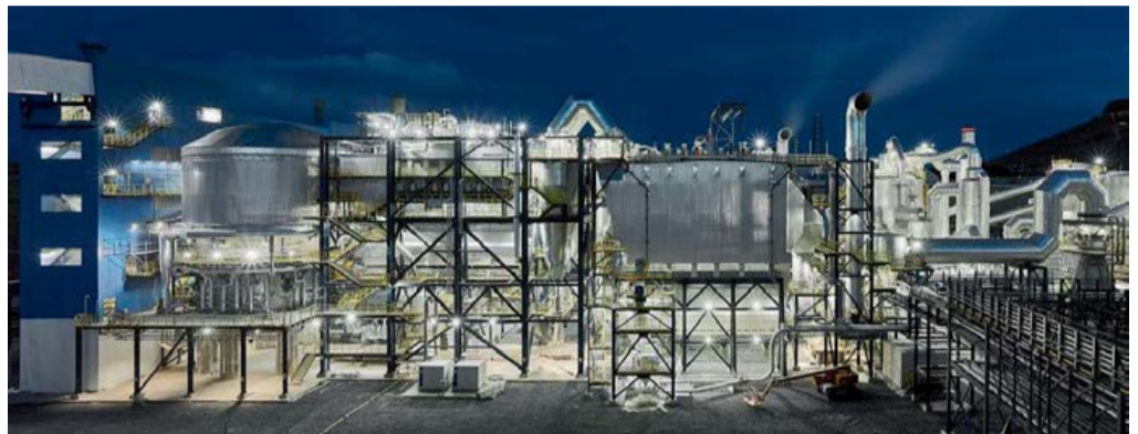
Mazidagi's roasting-gas cleaning-acid plant sections.
