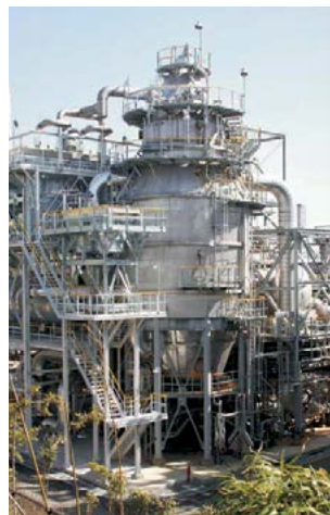
Fig. 4: Ammonium sulphate reactive crystalliser. PHOTO: GEA
