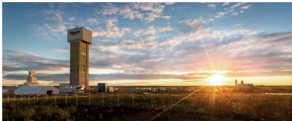
Mosaic is ramping up production at its Esterhazy K3 mine expansion.
