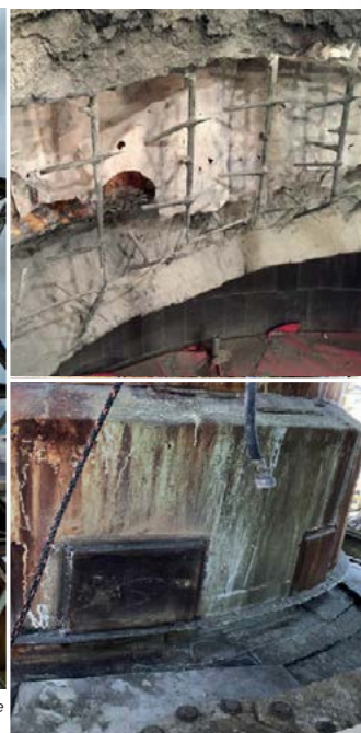
View of upper part of quench tower before replacement (above); damage to inside and outside of quench tower before replacement of upper part (right).
