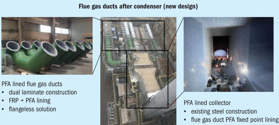
Fig 8: Overview of the new flue gas duct system
