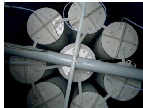
Fig. 8: WSA candle filters with wetting ring system.
