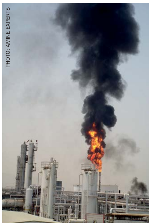
Fig. 1: Sour hydrocarbon-rich flare gas.
