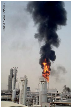
Fig. 1: Sour hydrocarbon-rich flare gas.
