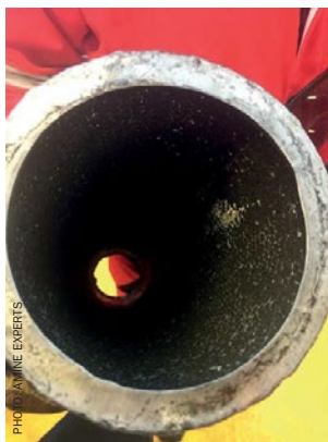
Fig. 10. Suction strainer plugged by particles from the amine solution.
