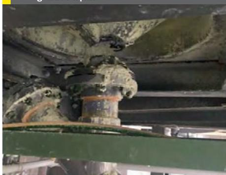
Fig. 3: Temporary repairs to scrubber outlet duct
