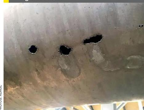
Fig. 2: Bottom of stack completely corroded at sulphur granulation plant
