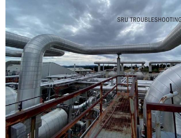
Direct fired reheater outlet line to the downstream converter.
