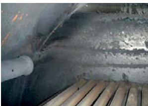
Fig. 6: Blowdown collection lateral
