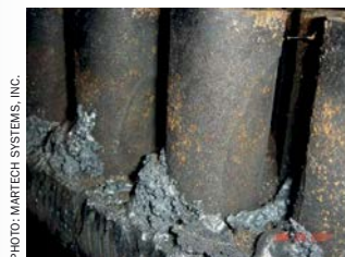
Fig. 1: FAC on condenser inlets (high purity BFW)
