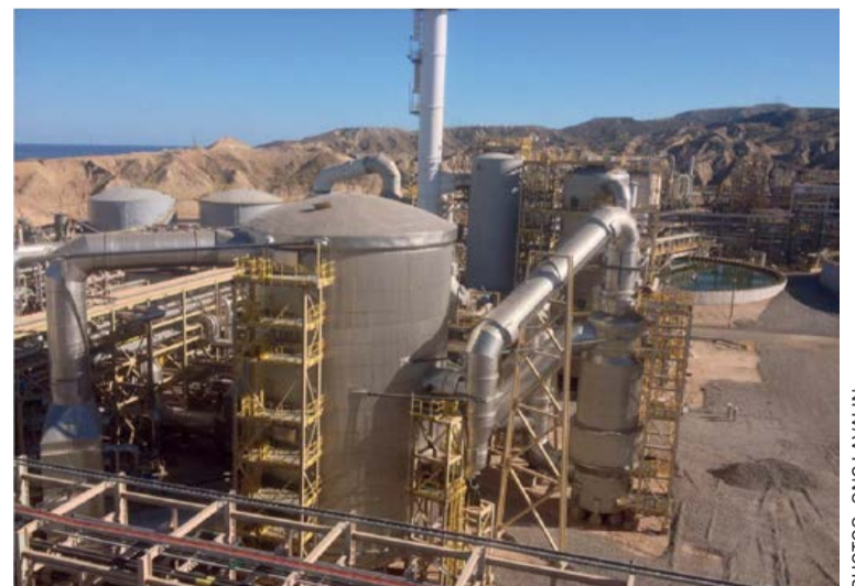
A sulphuric acid plant with HRS in a hydrometallurgical complex.
