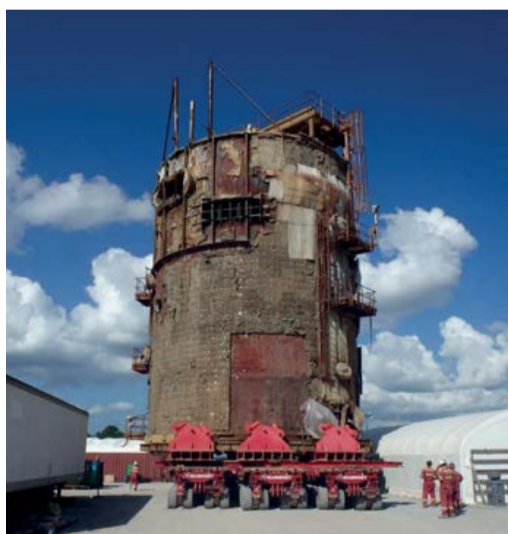
Fig. 7: Demolition and wheel out (left) and wheel in of new converter (right).
