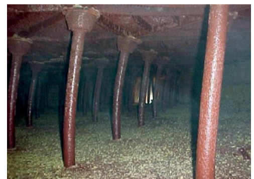
Fig. 3: Failing posts.
