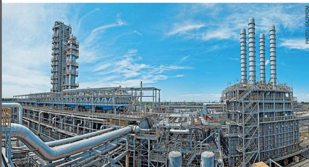
The Astrakhan gas processing plant.
