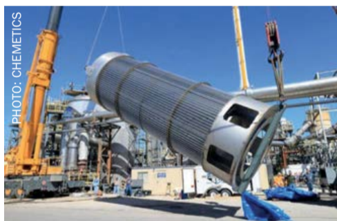
Fig. 10: New HHX prepared for installation as complete unit.
