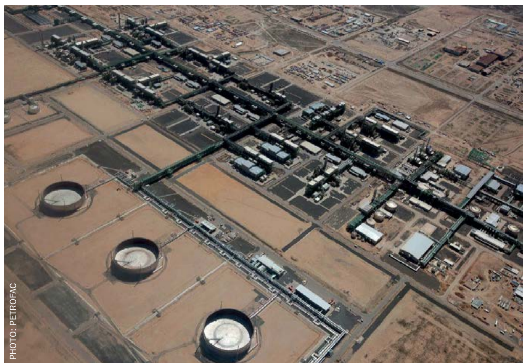
Onshore facilities at Kashagan.
