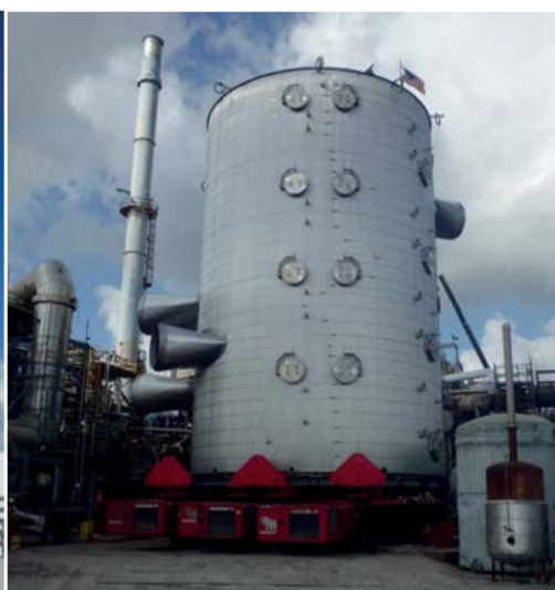
Fig. 7: Demolition and wheel out (left) and wheel in of new converter (right).
