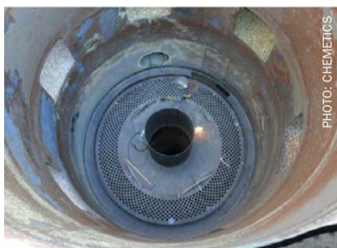
Fig. 8: Exposing top of internal HHX for removal.
