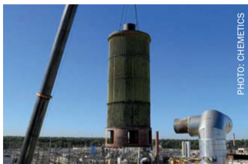
Fig. 9: Removal of old HHX complete unit.
