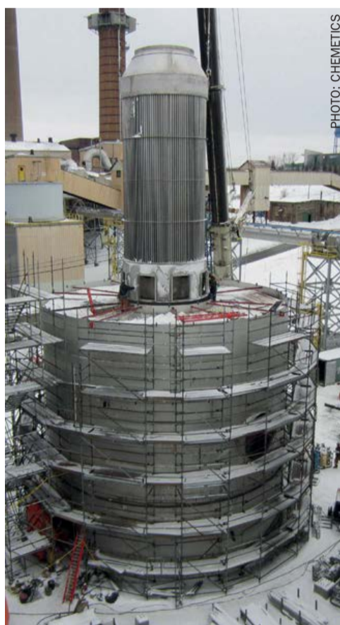
Fig. 6: Installation of internal gas exchanger.
