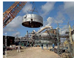
Fig. 14 (above left): Complete level lifted into position. Fig. 15 (above right): Dimensionally stable module completed at chemetics fabrication facility.
