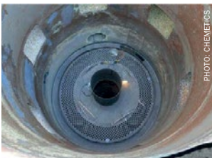
Fig. 8: Exposing top of internal HHX for removal.
