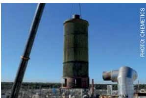
Fig. 9: Removal of old HHX complete unit.
