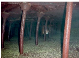
Fig. 3: Failing posts.
