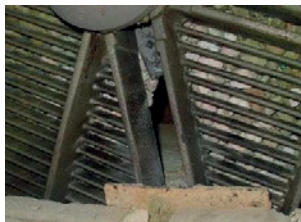
Fig. 3: Failing posts.
