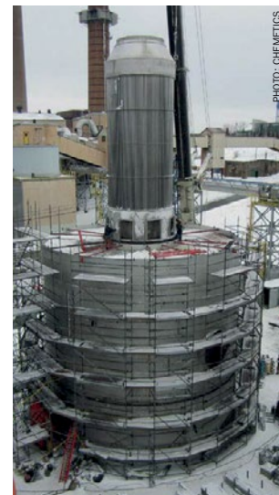
Fig. 6: Installation of internal gas exchanger.
