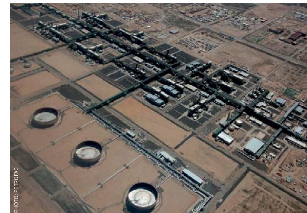
Onshore facilities at Kashagan.
