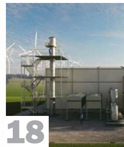
18 Cryogenic storage Addressing the intermittency challenges of renewable energy
