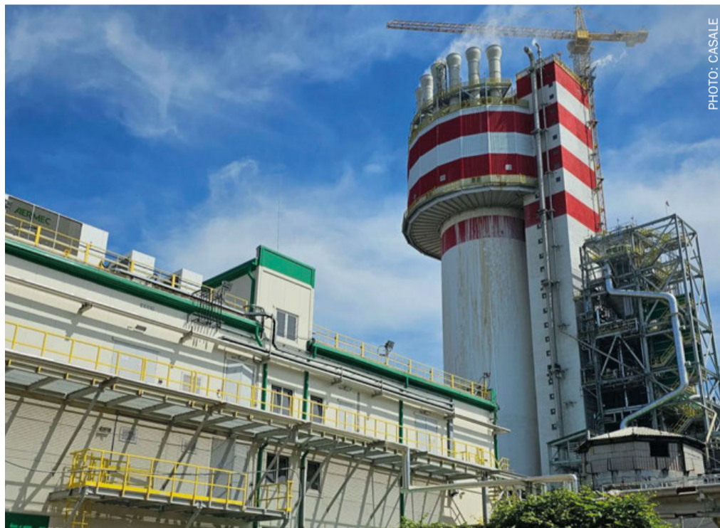
Togliatti's newest urea unit, commissioned in 2022.
