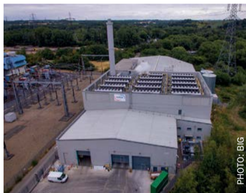
The Bioenergy Infrastructure Group (BIG) waste gasifier at Hoddesdon, near Hull, UK; a failed gasification project.
