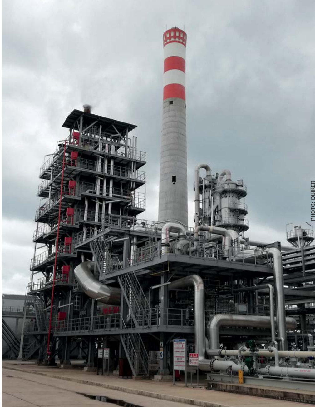
Fig. 2: SCO unit in a refinery in Asia.
