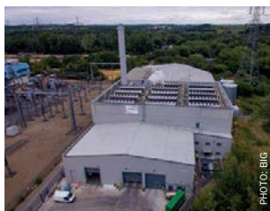
The Bioenergy Infrastructure Group (BIG) waste gasifier at Hoddesdon, near Hull, UK; a failed gasification project.
