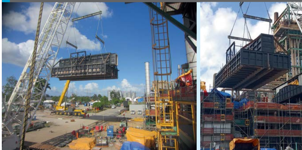
Fig. 4: Upper hood of the convection section
