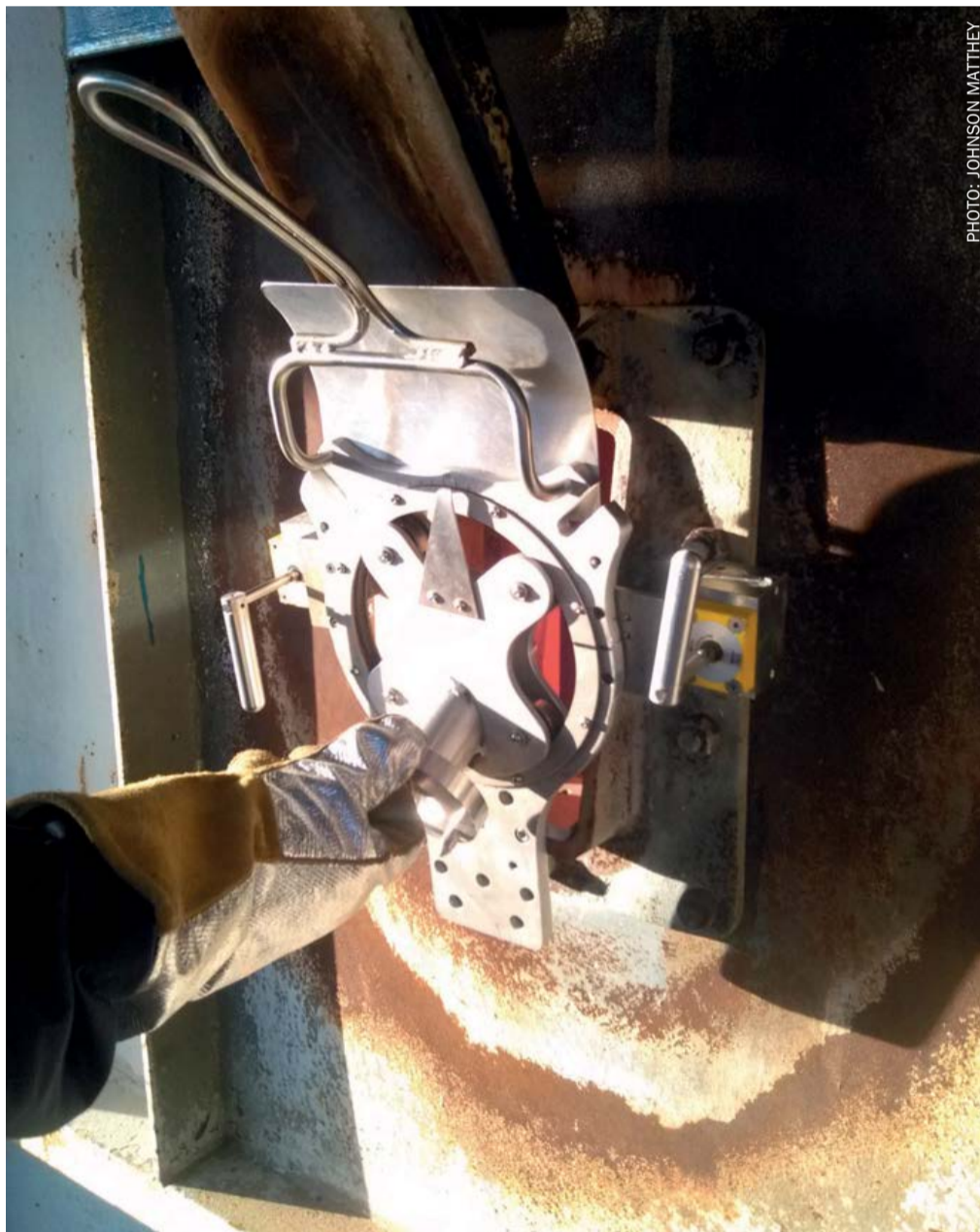
Fig. 9: Photo of Reformer Imager clamp in use on reformer peephole at Yara Le Havre.
