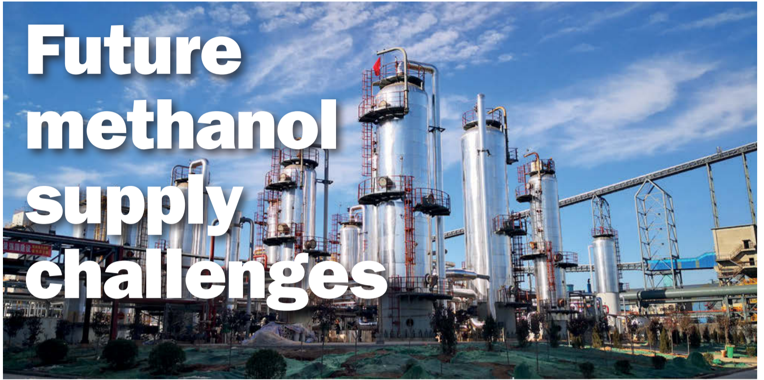
Above: CRI's new 110,000 t/a carbon capture methanol plant, Anyang, China.
