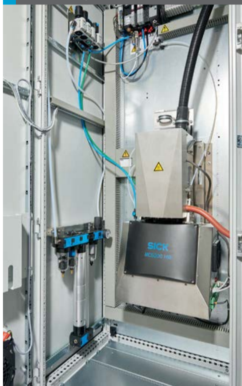
Fig. 2: MCS 200 HW hot extractive analyser
