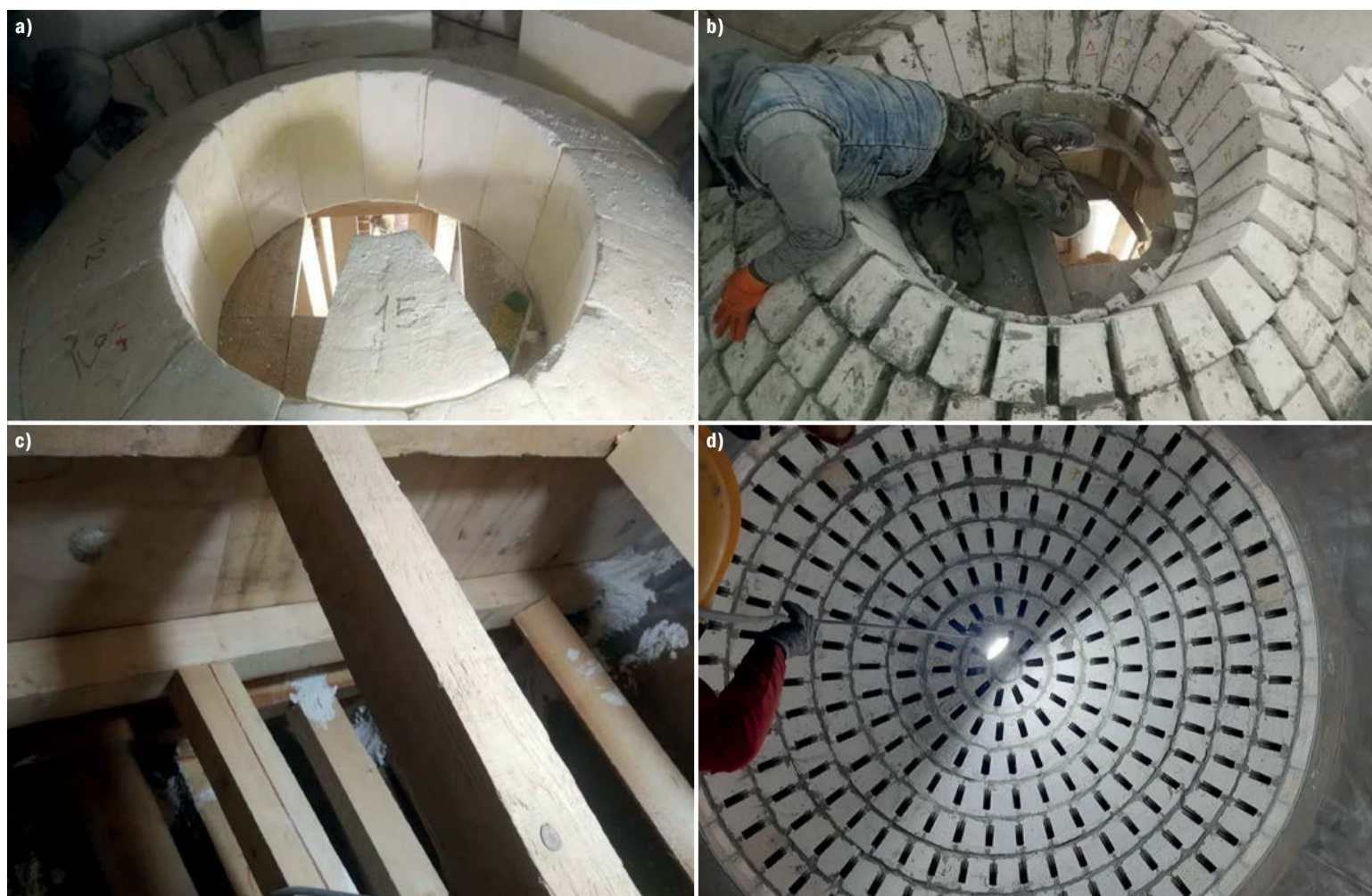
Fig. 11: a) View of polystyrene forms; b) Installation of dome bricks; c) View of wooden beams and probes; d) Final dome brick from bottom view.
