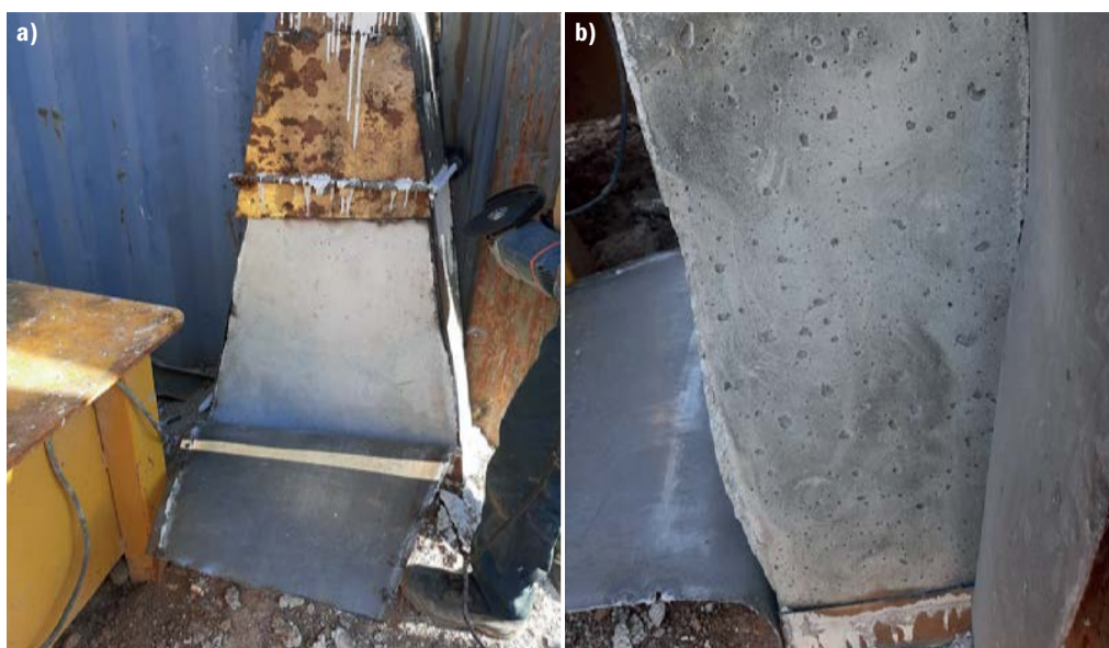
Fig. 4: Mock-up test a) General view of mock-up sample and cutting the form after casting; b) Side view of sample.
