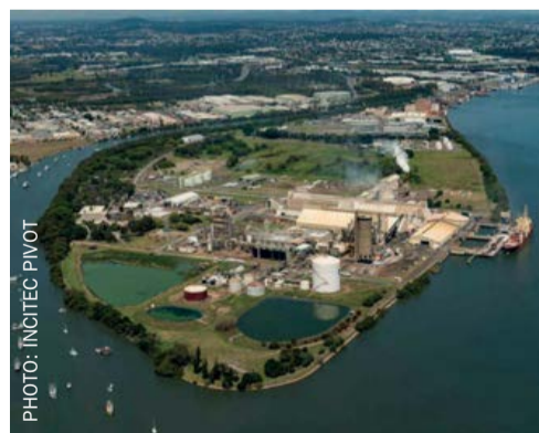
Incitec Pivot’s Gibson Island plant, Australia.
