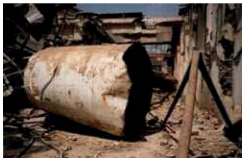
Fig. 1: Front of the tank.
