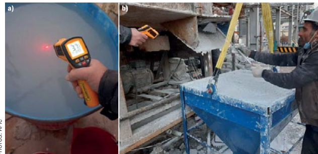
Fig. 6: a) Measuring the temperature of water; b) Pouring refractory into the hopper.
