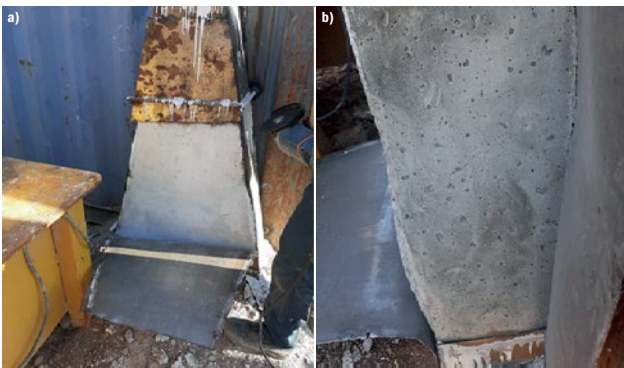
Fig. 4: Mock-up test a) General view of mock-up sample and cutting the form after casting; b) Side view of sample.
