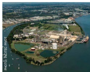
Incitec Pivot's Gibson Island plant, Australia.
