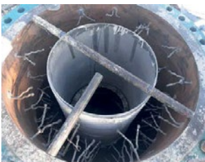
Fig. 2: View of welded anchor bolts and their cellulose acetate caps.
