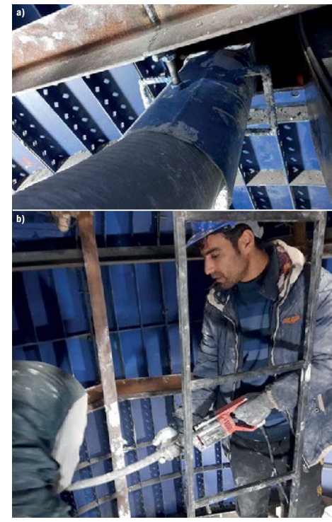
Fig. 9: a) Draining the casting material into the opening of forms through a flexible hose and chute; b) Internal vibrator via the window opening.
