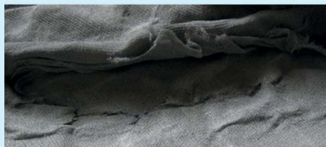
b) Cracking due to thermal stresses
