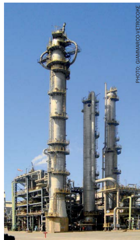
GV low-energy CO 2 removal unit.
