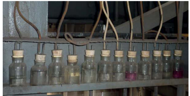
Fig. 1: A typical passive leak detection system.
