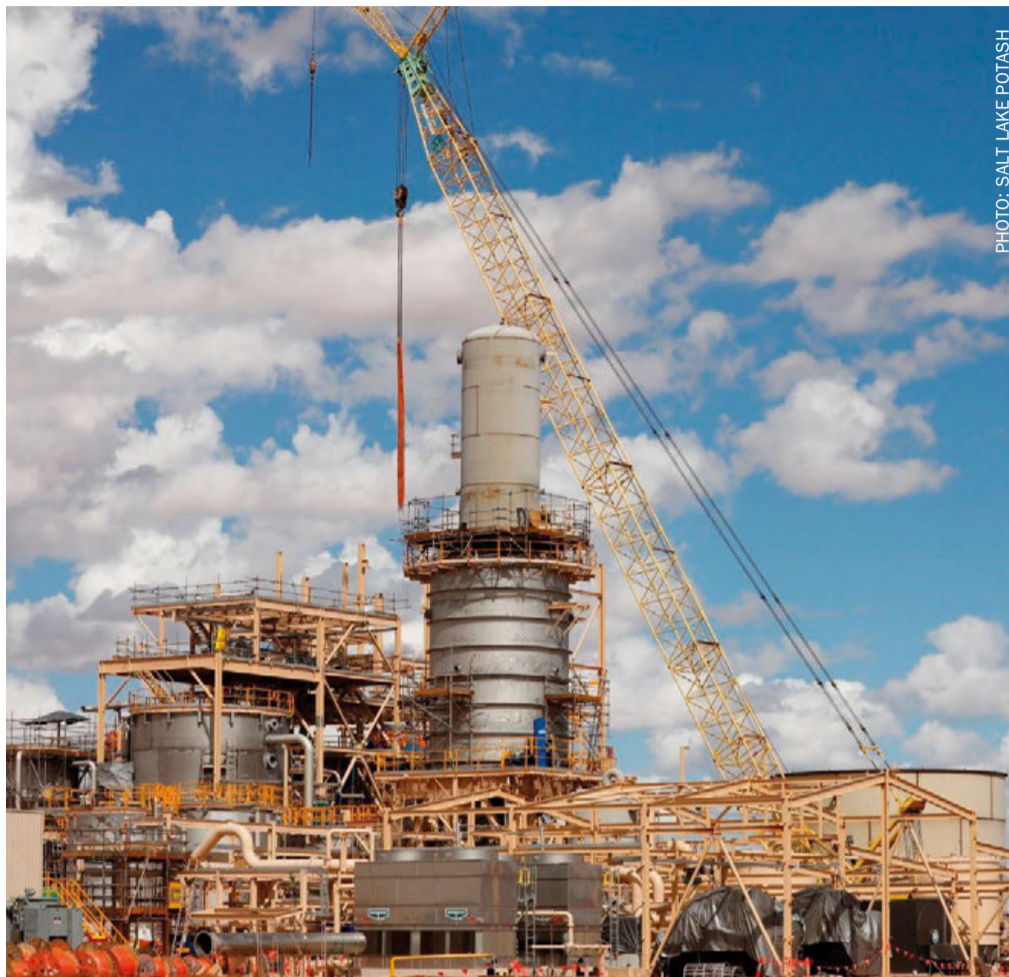
Erection and installation of the SOP crystallisation plant at Lake Way, Western Australia.
