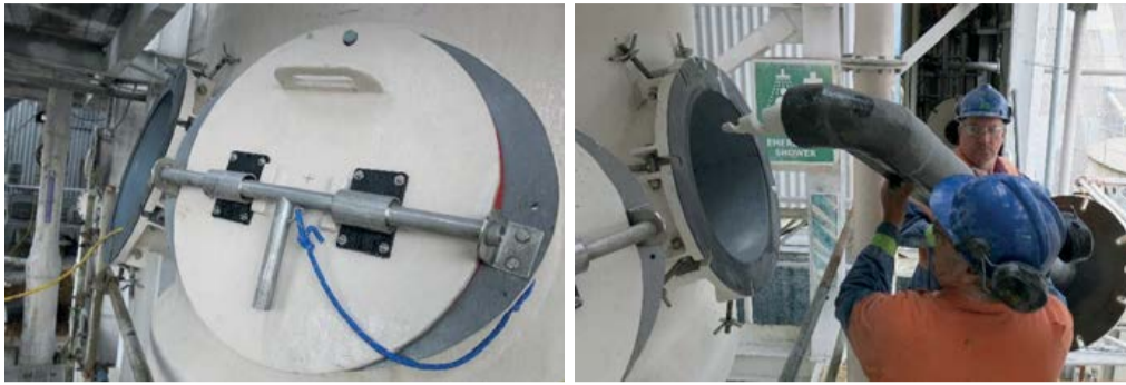
Quick release access hatches (left) provide fast and safe access for inspection and maintenance. Clever design (right) allows maintenance to be done without confined space entry.
