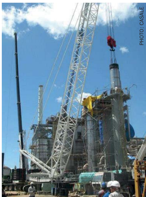
Casale's revamp of the CF Braun ammonia plant focused on the reduction of carbon dioxide emissions.
