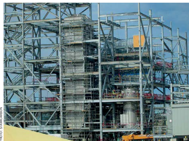
The granulator, quench vessel and advanced MicroMist™ Venturi (MMV) scrubbing system installed at DGC's Beulah urea plant in North Dakota.
