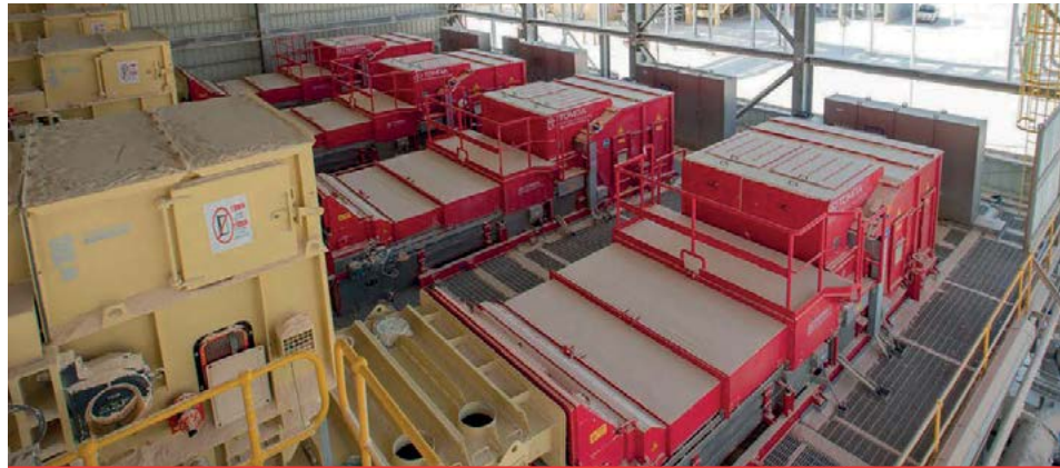
An array of four TOMRA sorting machines at the MWSPC mega project in Saudi Arabia.
