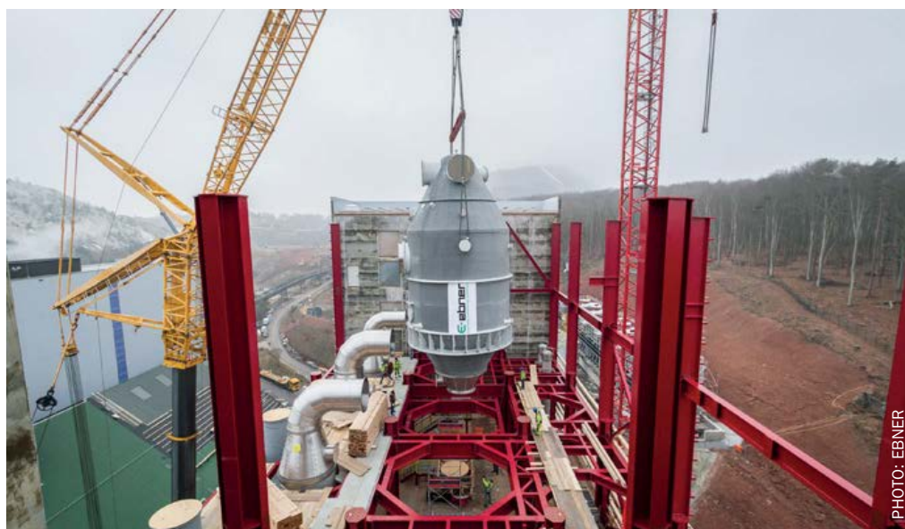
Ebner designed, manufactured and erected this evaporation and crystallisation plant for K+S.
