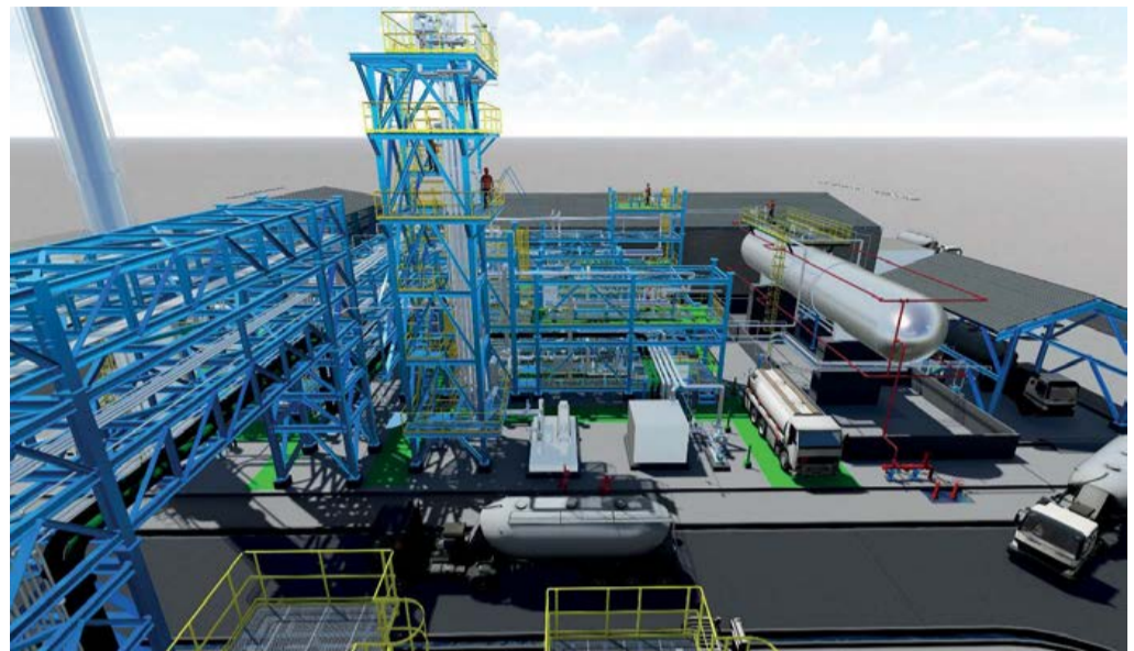
Fig. 1: Example of a thyssenkrupp Uhde small-scale modular green ammonia plant showing ammonia synthesis (centre) and pressurised ammonia storage tank (right).
